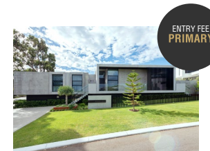
New Residential Buildings (over $3.0m)
